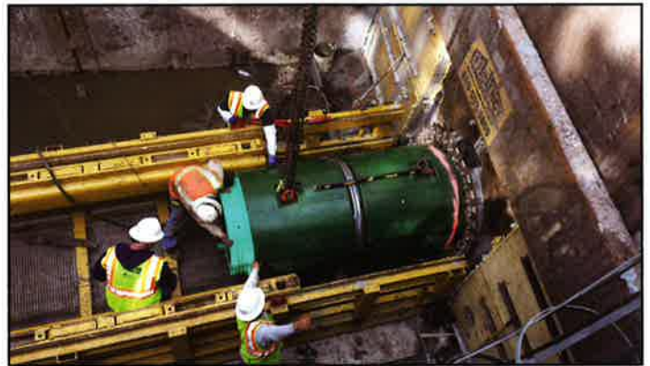
Launching of Huxted MTBM at Sun City Center in Florida.
